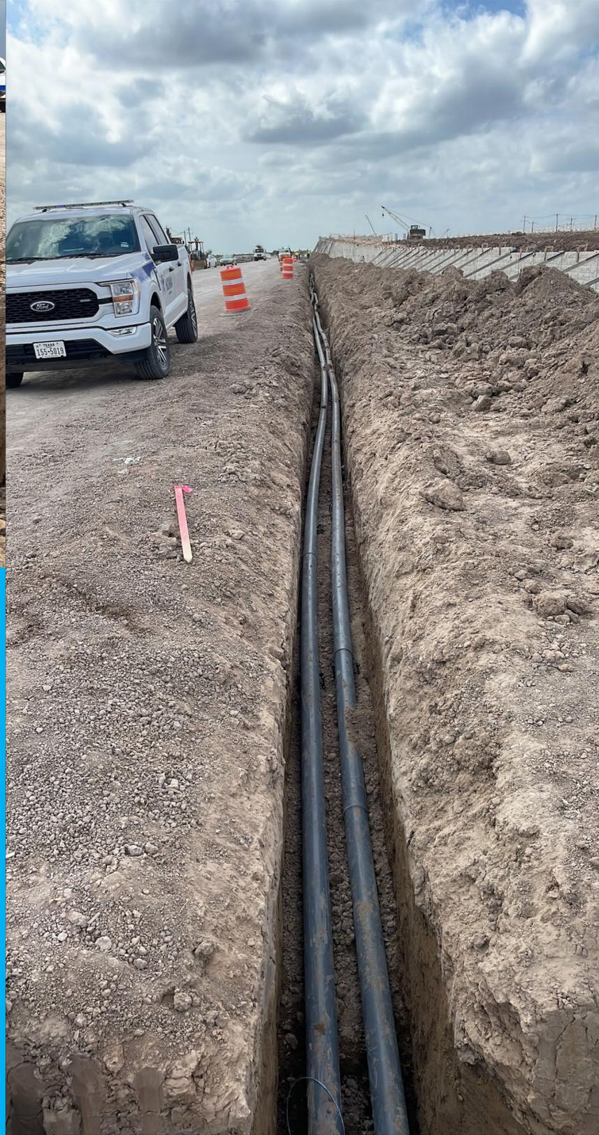
Trenching and installation of conduit for toll collection system hardware.
