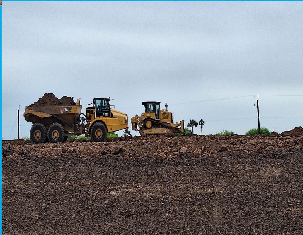
Placement \delivery of flexbase material to the East side of San Juan Canal embankment
