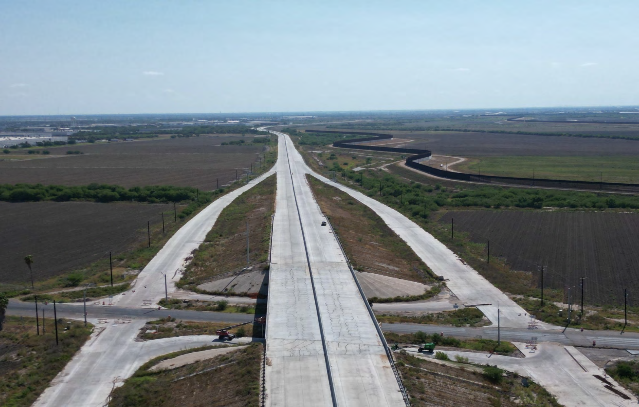
FM494 [Shary Bridge Slab]
