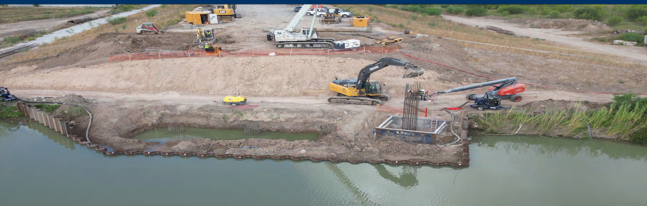
San Juan Main Canal Bridge East / West
