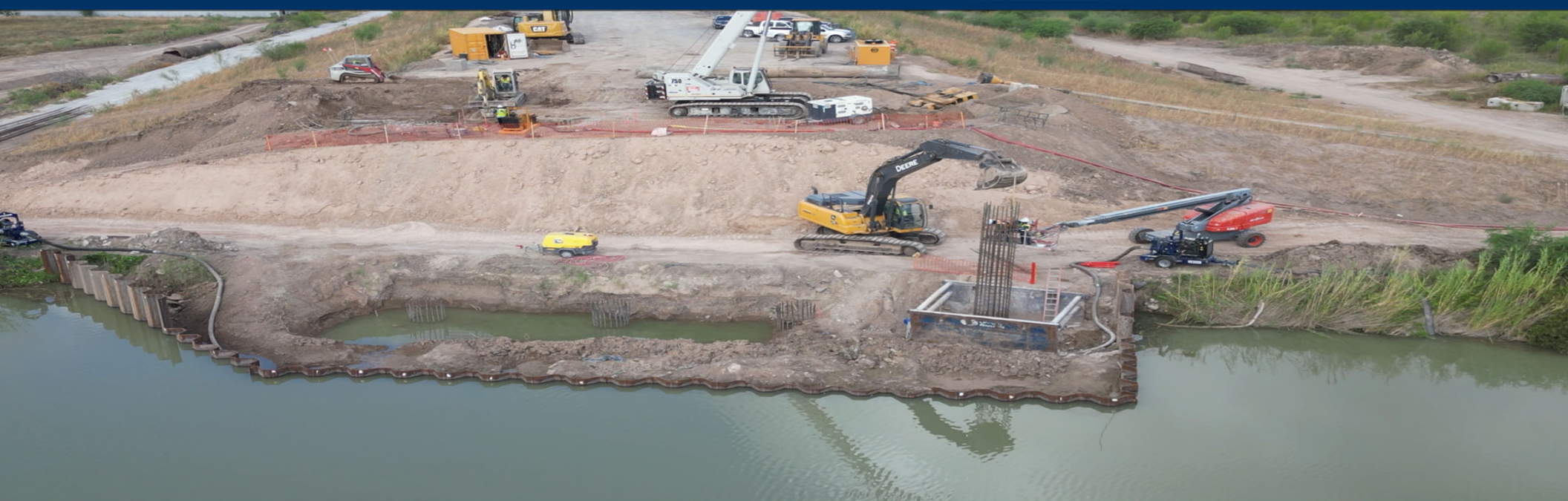
San Juan Main Canal Bridge East / West
