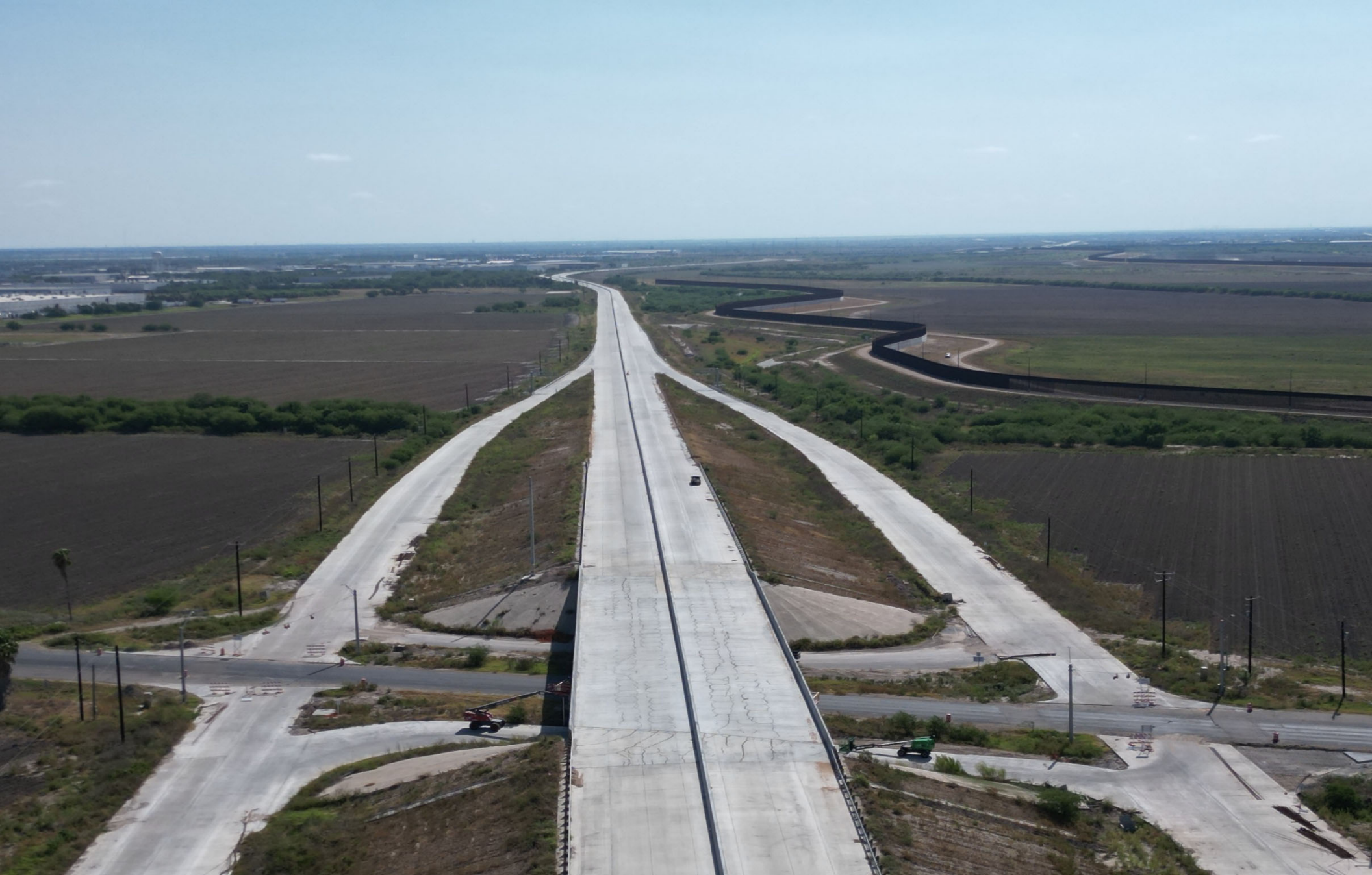
FM494 [Shary Bridge Slab]
