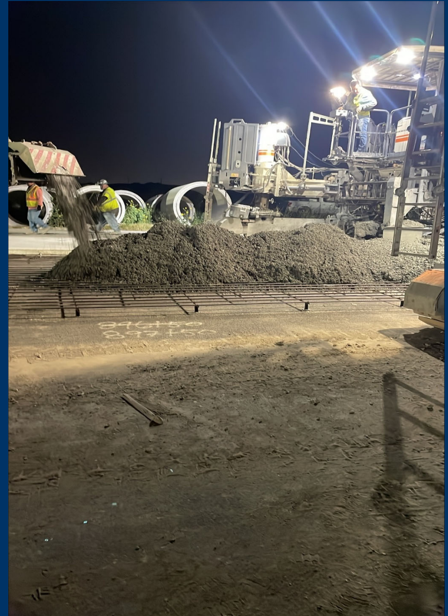
CEMENT TREATED BASE / CONTINUOUSLY REINFORCED CONCRETE PAVING
