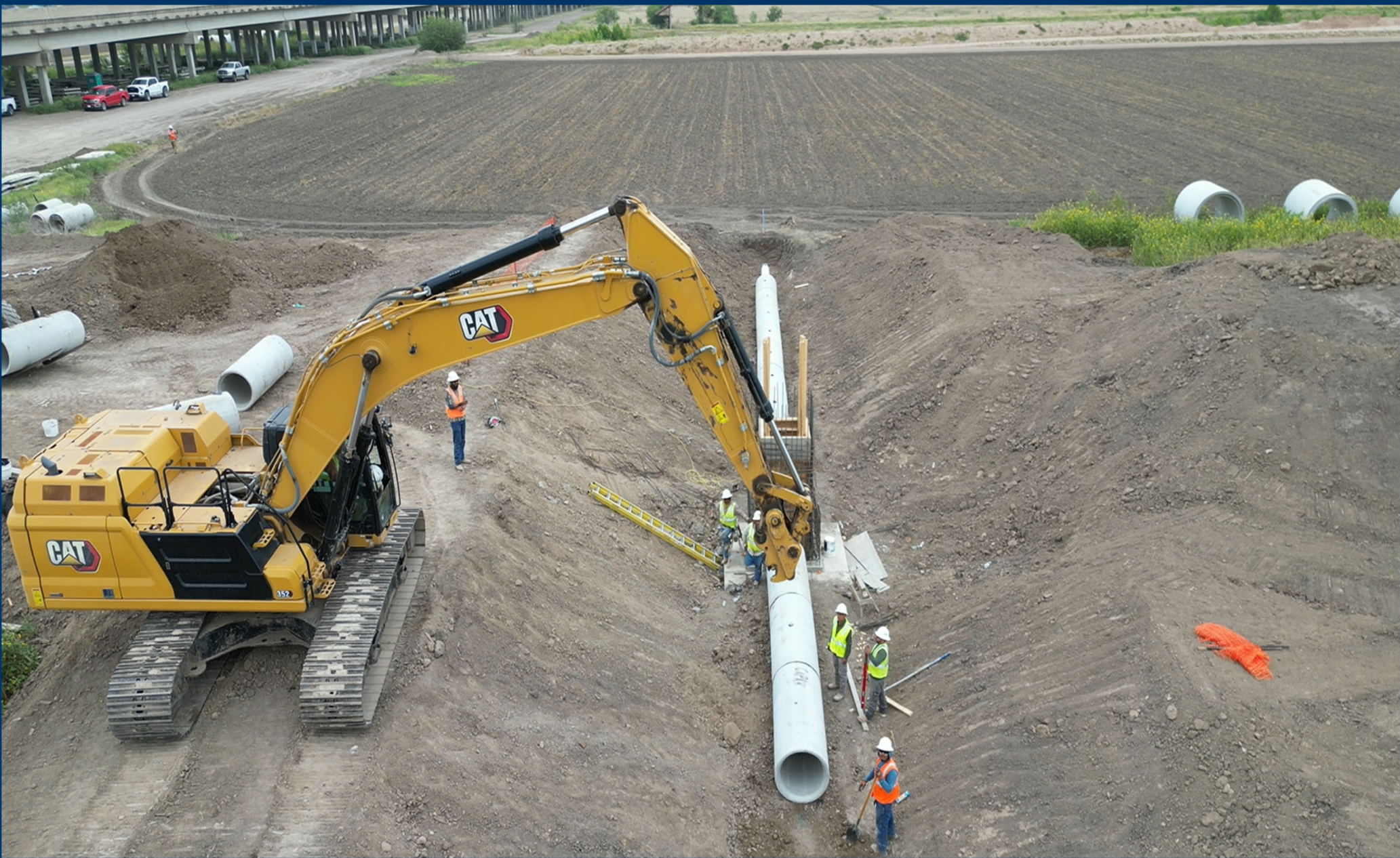
Irrigation Structure at STA. 1024+00
