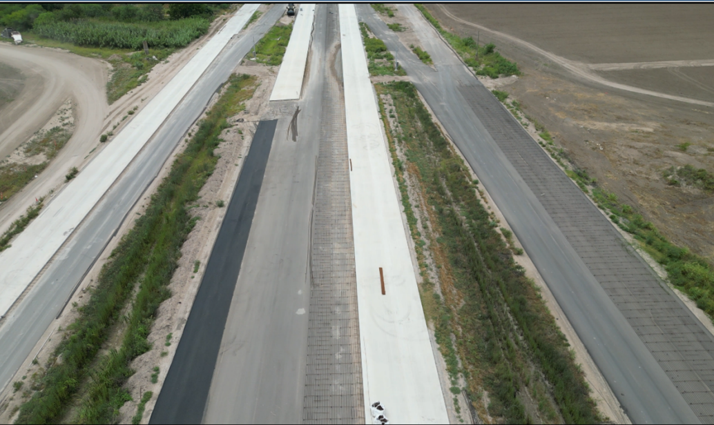
CEMENT TREATED BASE / CONTINUOUSLY REINFORCED CONCRETE PAVING
