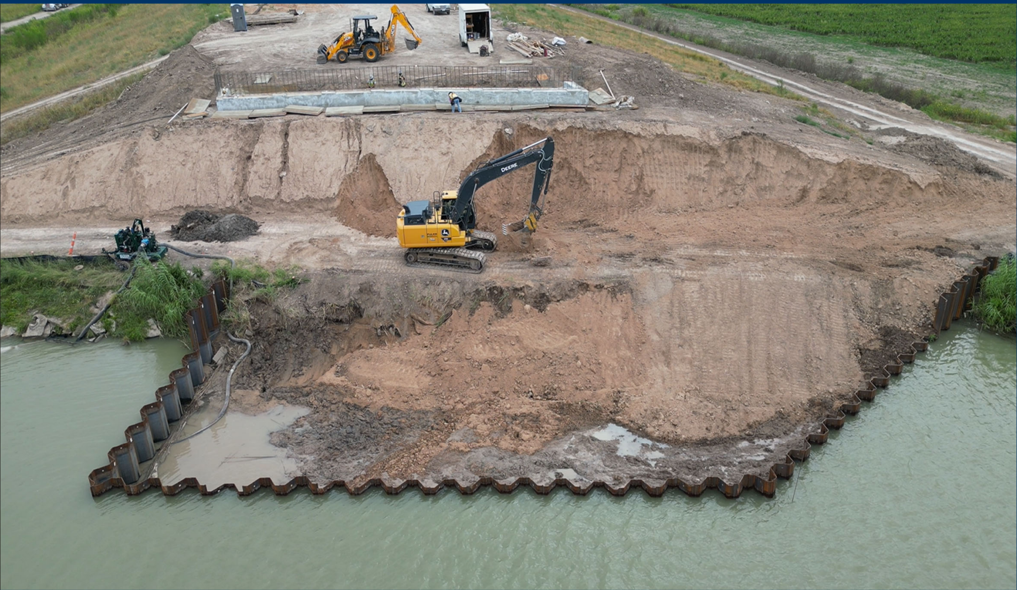
San Juan Main Canal Bridge BENT 3
