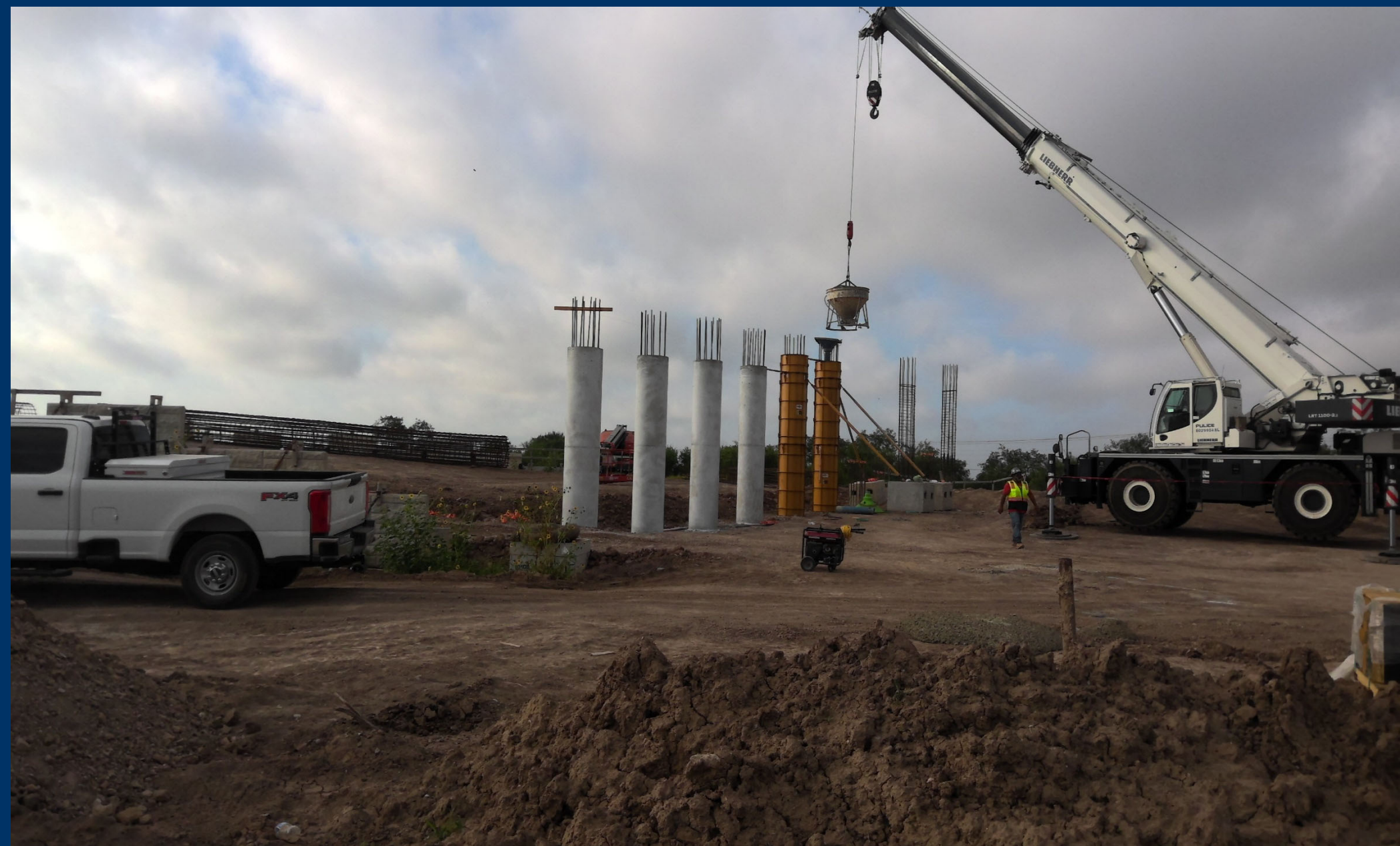
Drill shafts / columns on Abutment 2 of Jackson Overpass
